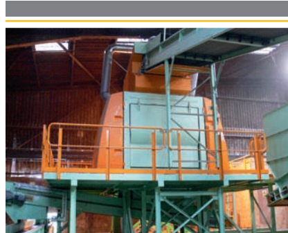
Application: Industrial and commercial waste Solution: TR3200 Location: Great Britain
